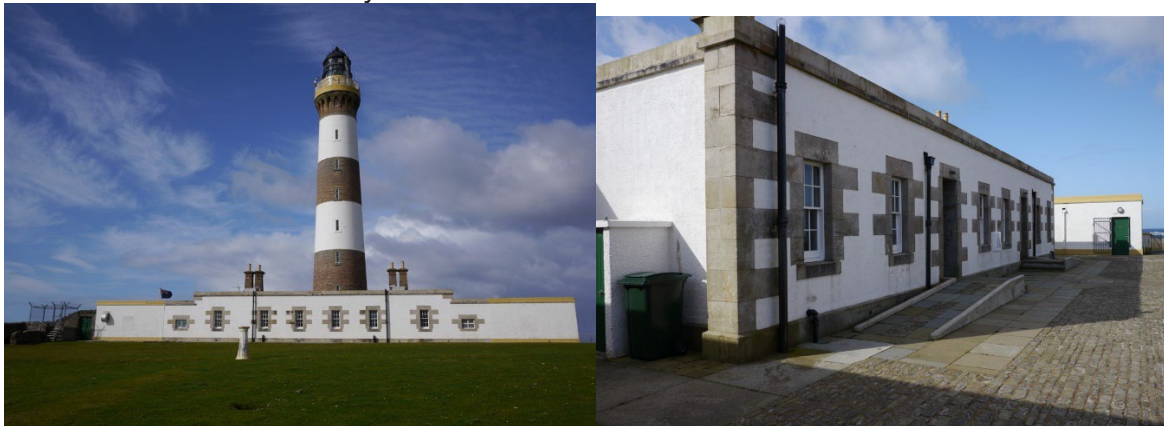
Figure 3 Lighthouse Keeper’s Cottages, Exterior
