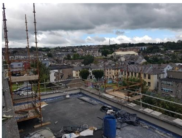
Figure 29: Maintenance work in progress, refelting on one of the principal flat roof sections over the altar – Image © NCE Insulation
