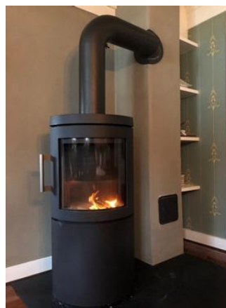
Figure 54: The GSHP is supplemented by a wood burning stove – Image © Landsverk
