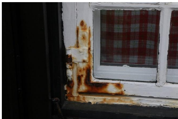
Figure 51: Pre-retrofit, deterioration of existing window frames – Image © Landsverk
