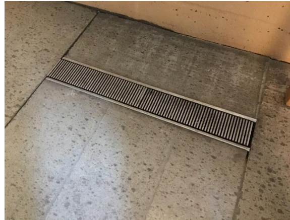
Figure 46: Warm air input vent, corresponding extract vents appear adjacent to the opposite wall in the main space – Image © Historic Environment Scotland – Photographer: Kenneth Easson
