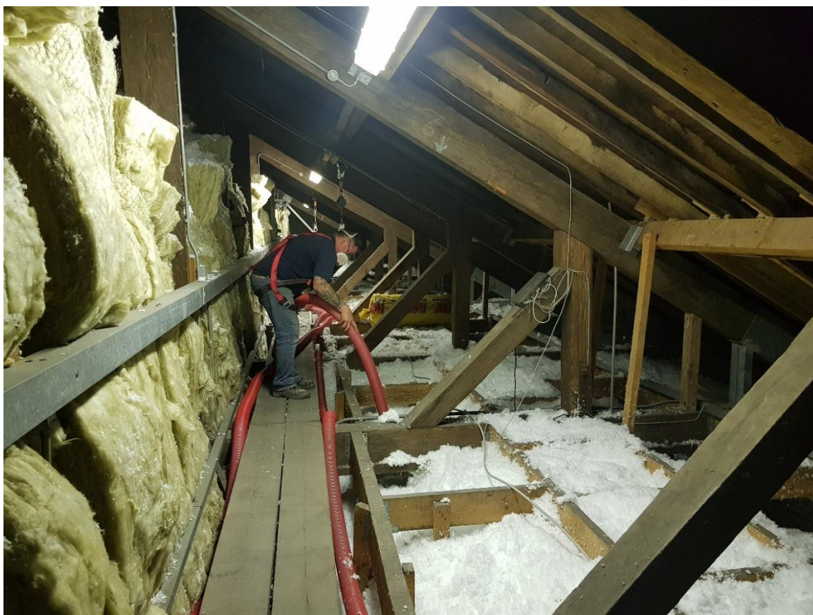
Figure 28: Insulation installation in the cathedral pitched roof during 2021 – Image © NCE Insulation
