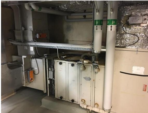
Figure 45: Warm air system plant room, also mixes pre-heated fresh air with recirculated air to provide ventilation – Image © Historic Environment Scotland – Photographer: Kenneth Easson
