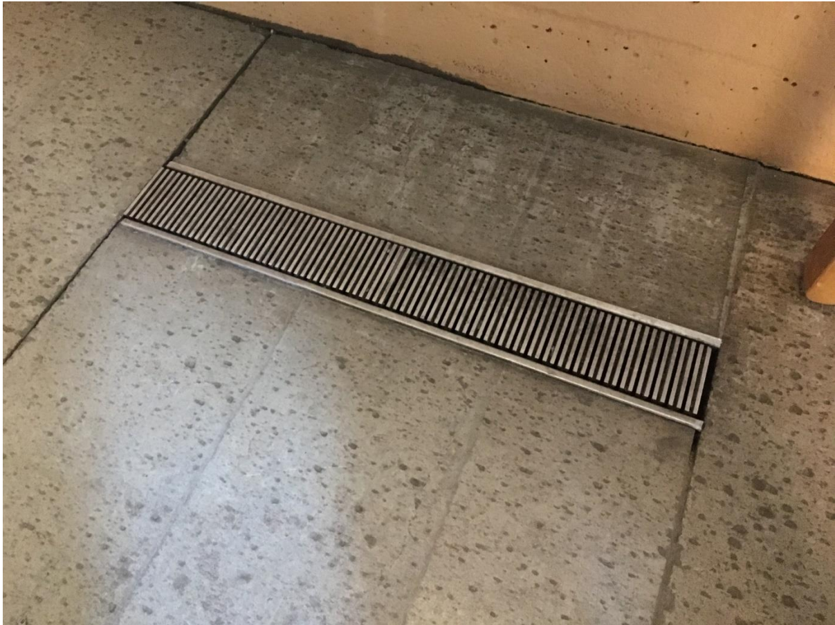
Figure 15: Input vent from the mechanical ventilation system adjacent to the northeastern external wall – Image © Historic Environment Scotland – Photographer: Kenneth Easson
