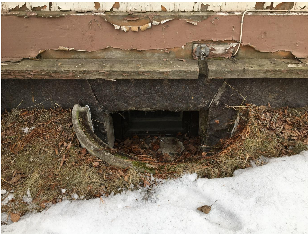
Figure 9: Modern semi-circular concrete ring added to protect an original ventilation opening, which has itself been modified to serve as a basement window – Image © Historic Environment Scotland – photographer: Kenneth Easson
