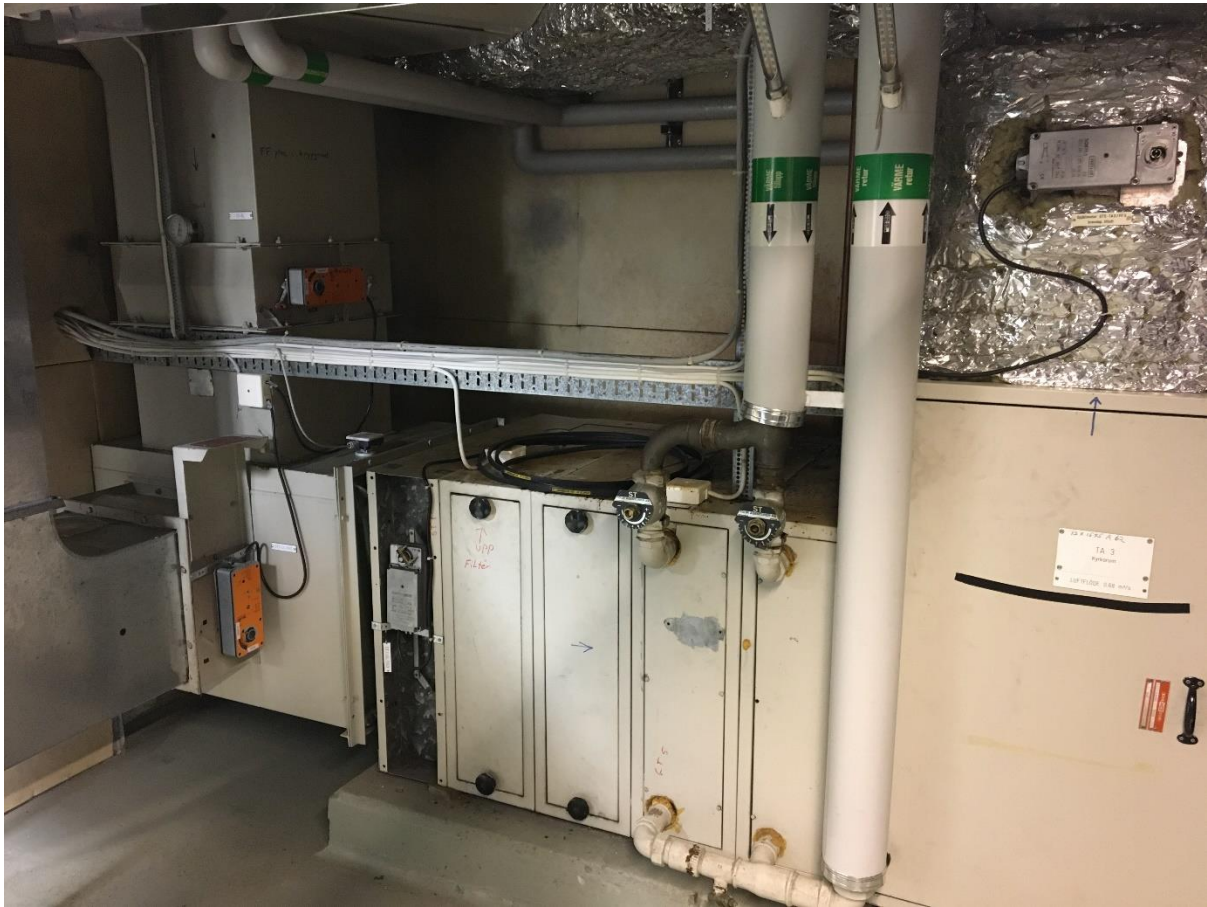
Figure 14: Heat recovery ventilation unit in the plant room at Tegn Church – Image © Historic Environment Scotland – Photographer: Kenneth Easson
