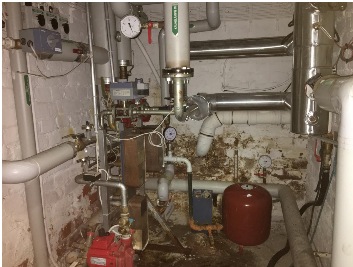
Figure 10: Basement room housing district heating plant equipment, note in particular the heat exchangers (three rounded metal cuboids to left of centre showing visible corrosion) – Image © Historic Environment Scotland – photographer: Kenneth Easson
