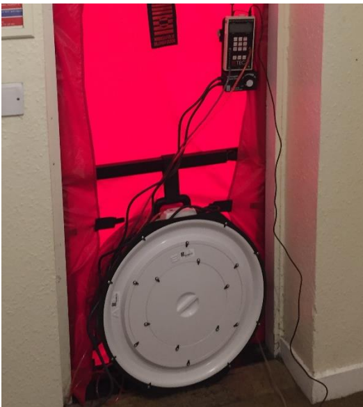
Fig 7. The fan installed in the sealed external door.
