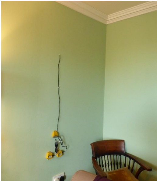
Fig. 2: Loggers measuring two points in this wall, at the top of the cable and nearer the loggers.
