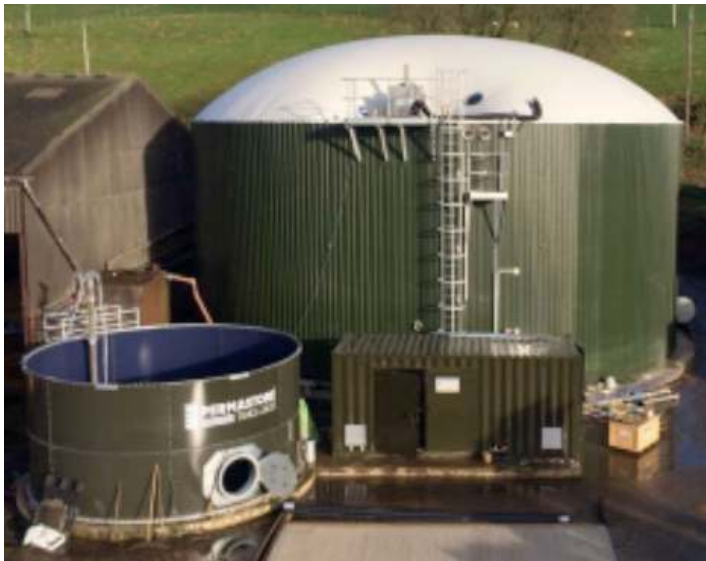
Right: Anaerobic digester generating biogas image from Agriland.ie
