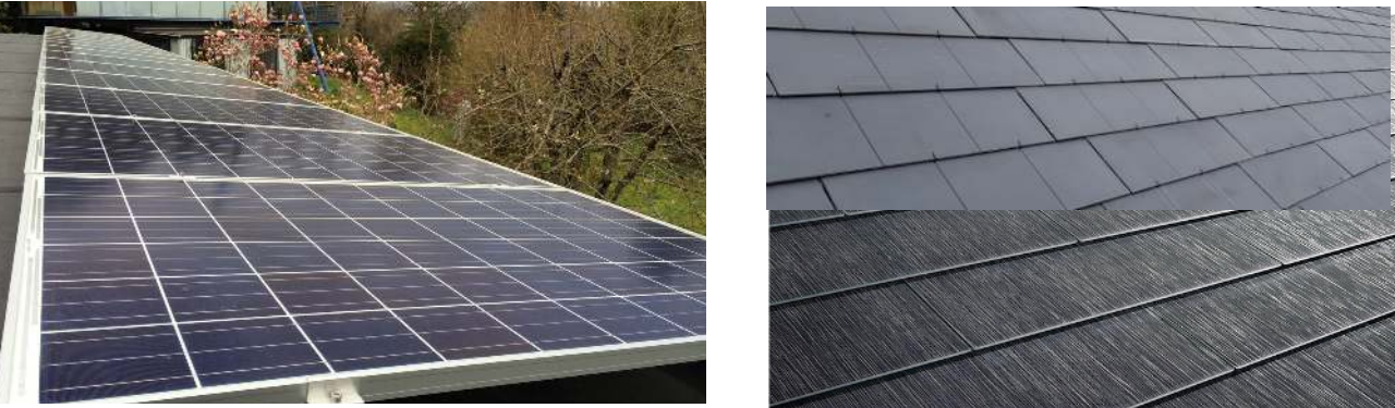
PV: Monocrystalline large panels 260Wp GB Sol slate effect above, Tesla glass tiles below
