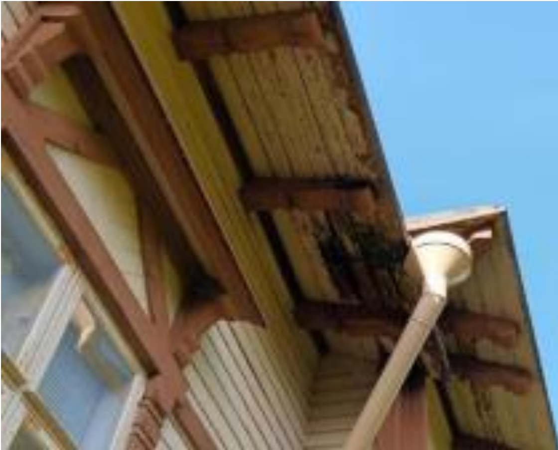
FIGURE 22. Leakage from the eaves on the lower surface and a new downspout (Riekki 2021)
