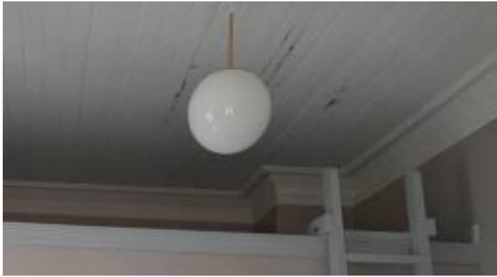
FIGURE 17. Moisture damage to the ceiling surface below the heat distribution room.
