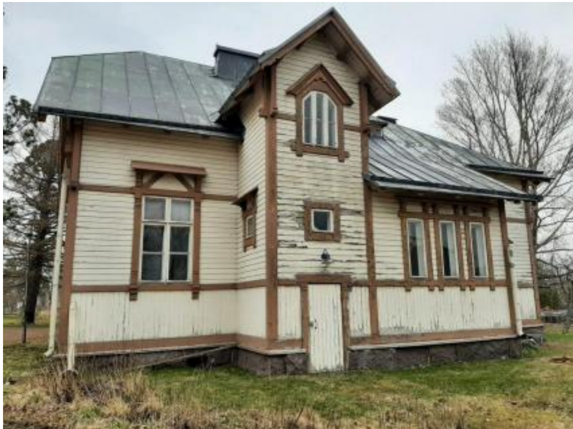
FIGURE 14. Significant deterioration of the end façade surface, a door leading to the basement near the ground and a fallen downspout on the left.
