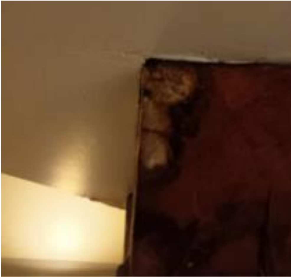
FIGURE 24. Leakage trace and signs of microbial growth at the base of the lattice (Riekki 2021)
