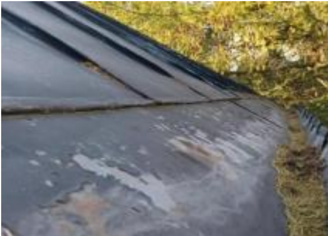
FIGURE 21. Paint and surface rust detached from the sheet metal roof and dirty footstool (Riekkı 2021)
