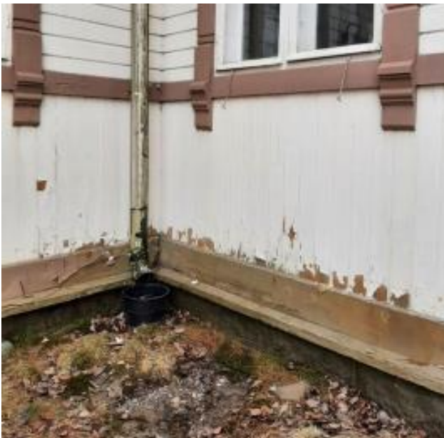
FIGURE 13. Damage to the lower part of the façade at the downspout
