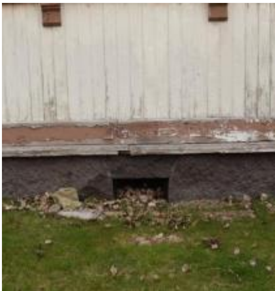
FIGURE 15. Basement ventilation hatch (Tolonen 2021)
