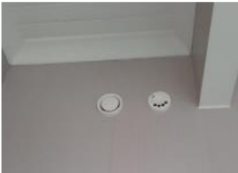
FIGURE 20. Side-by-side supply and exhaust air valves
