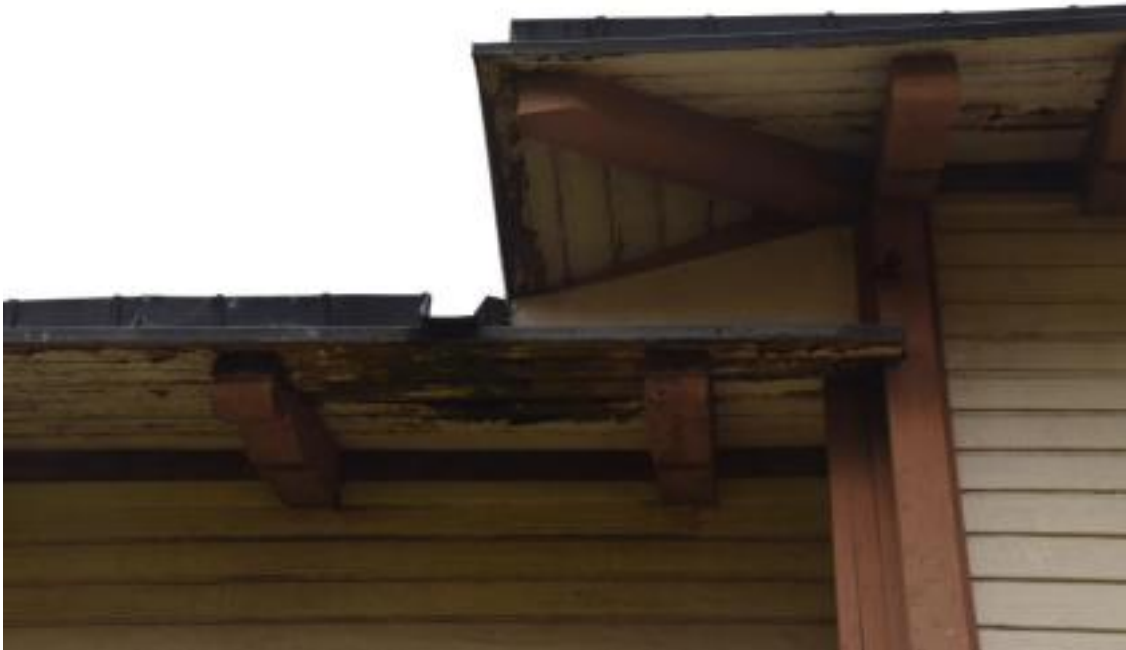
FIGURE 12. Damage to the underside of the eaves of the south-east façade (Tolonen 2021)
